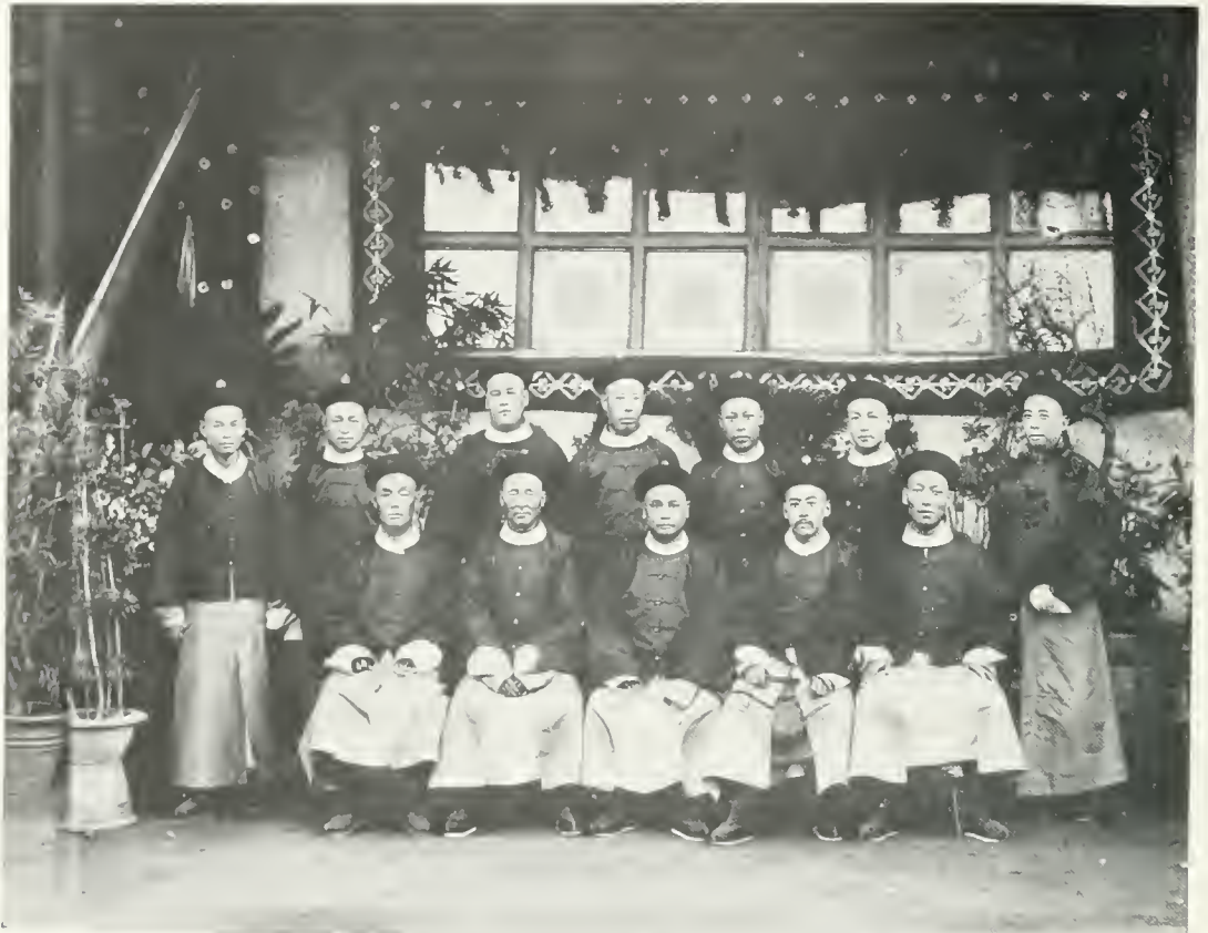
THE STAFF OF CHINESE OFFICIALS WHO BUILT THE PEKING-KALGAN RAILWAY. His Excellency Jeme Tien Yow, the engineer-in-chief, is in the centre.
