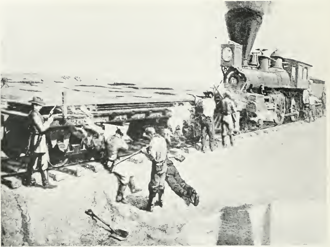
DEFENDING THE CONSTRUCTION TRAIN AGAINST THE SPIRITED ATTACKS OF HOSTILE RED INDIANS. An incident during the building of the first American transcontinental railway.
