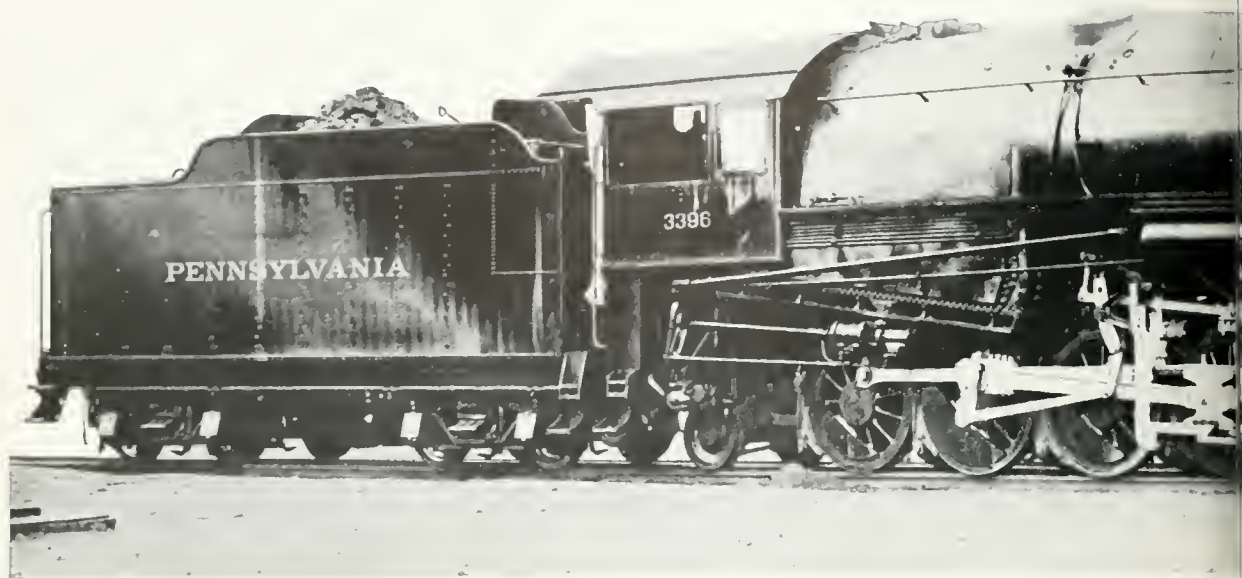
THE MAMMOTH MALLET ARTICULATED SIMPLE (2-8-8-2) LOCOMOTIVE USED This engine has 56-inch drivers; a total heating surface of 8,524.8 square
