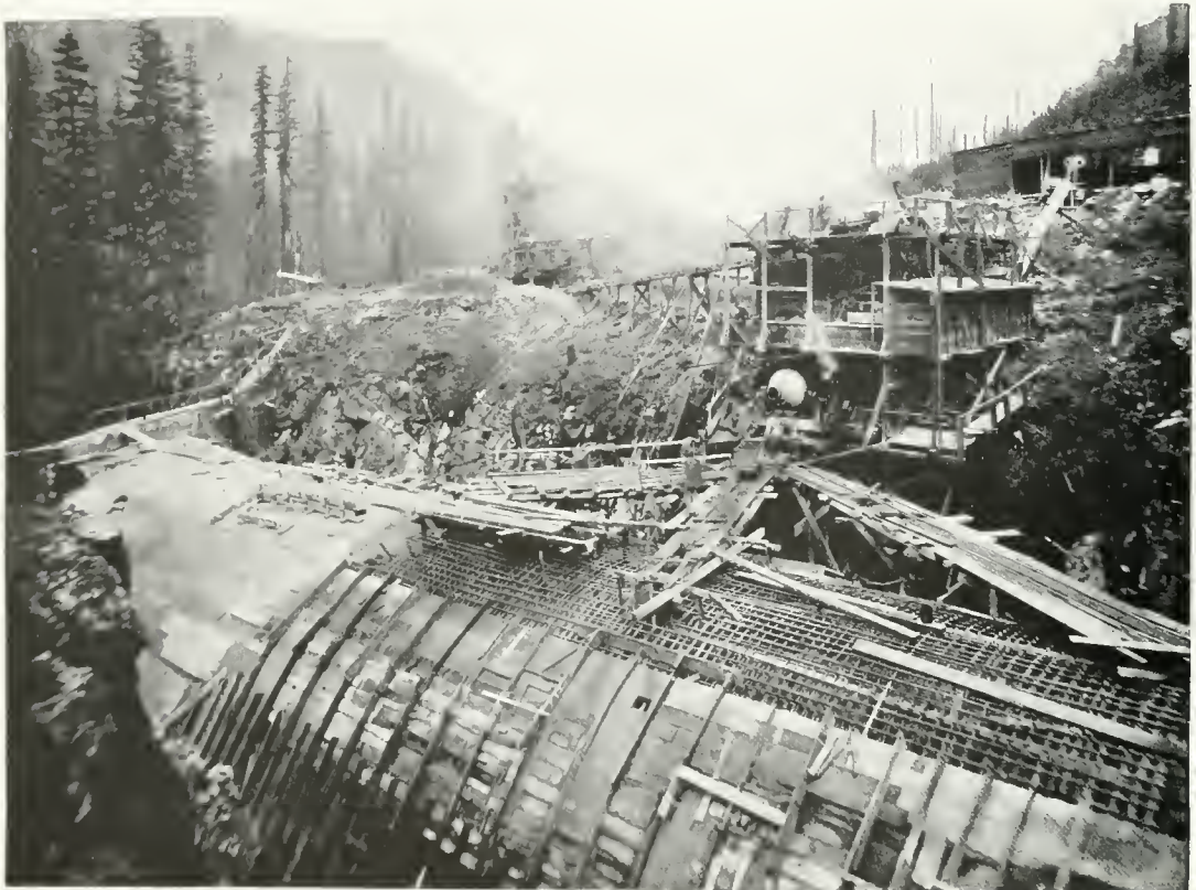
BUILDING THE PORTAL OF THE CASCADE TUNNEL.
