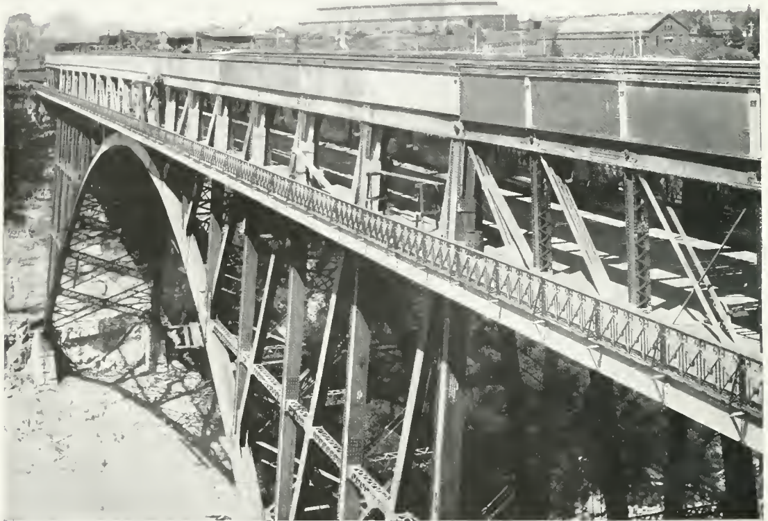
VIEW OF THE NIAGARA SPAN BRIDGE AFTER THE REMOVAL OF THE SUSPENSION BRIDGE. Showing top railway deck and lower deck for public use.
