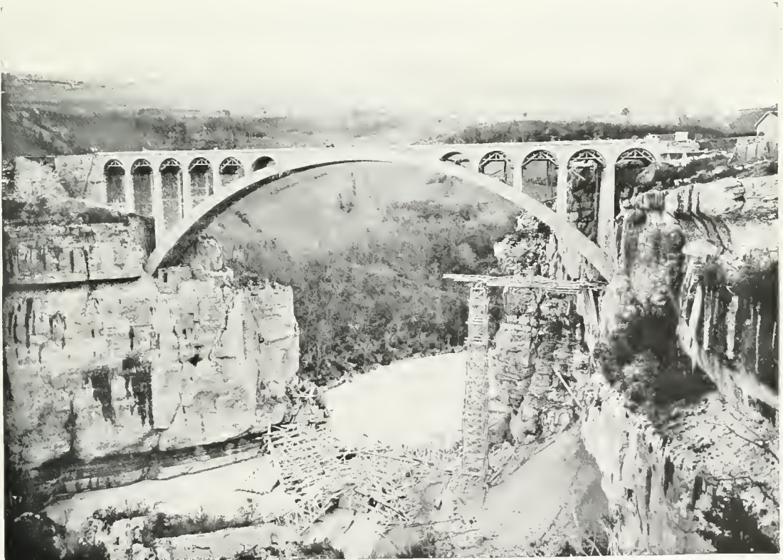
THE COMPLETED 267-FEET ARCH SPAN OF THE MONTANGAS MASONRY BRIDGE. Showing the timber falsework under demolition.
