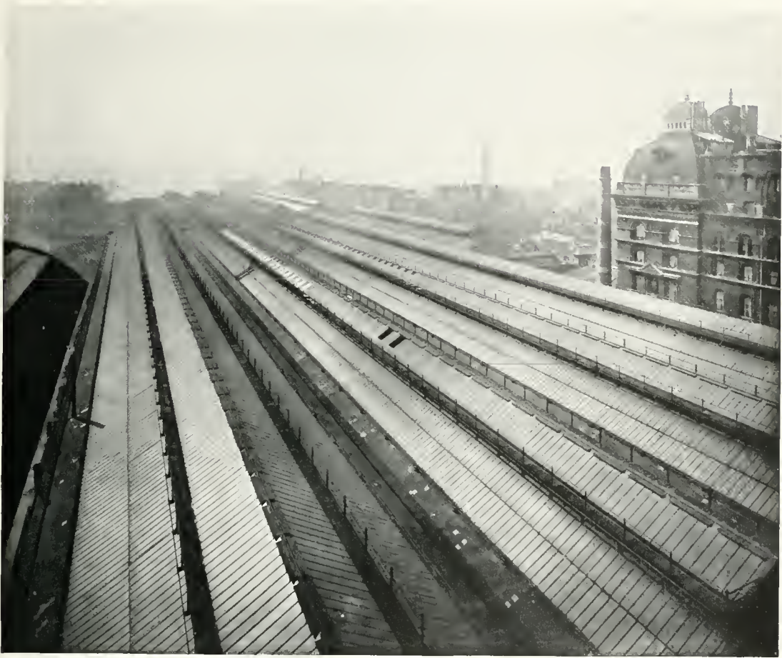
THE SEA OF GLASS FORMING THE ROOF OF THE NEW VICTORIA TERMINUS OF THE LONDON, BRIGHTON AND SOUTH COAST RAILWAY.
