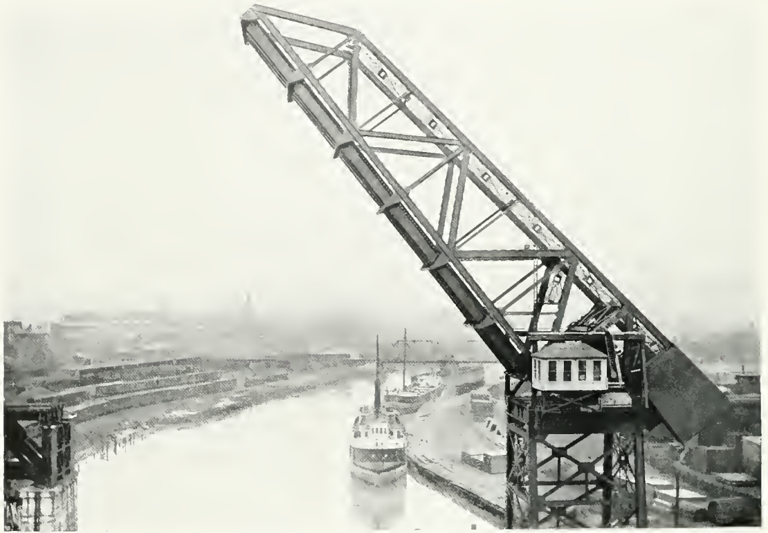
160-FOOT SINGLE-LEAF DOUBLE-TRACK SCHERZER ROLLING LIFT BRIDGE ACROSS THE CUYAHOGA RIVER AT CLEVELAND, OHIO, U.S.A.
