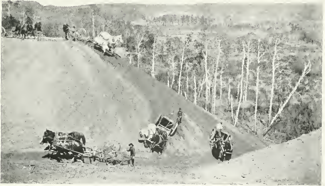
BUILDING A HIGH EMBANKMENT.
