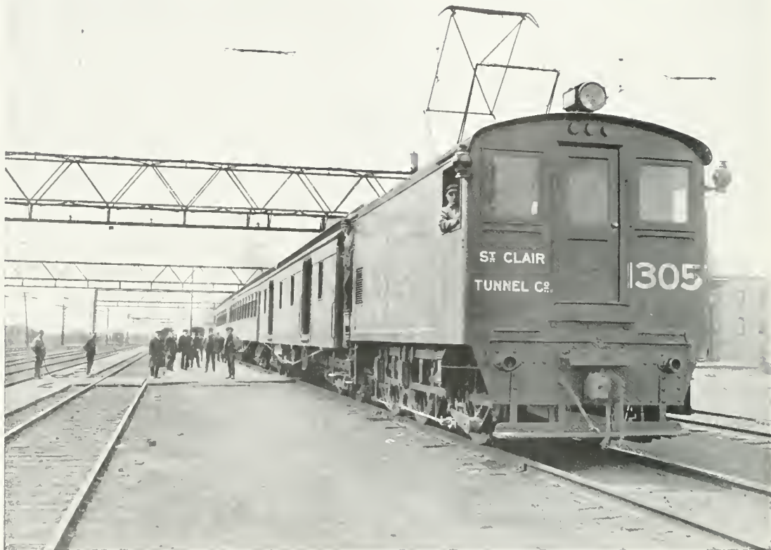
ONE OF THE ELECTRIC GIANTS WHICH "WORKS" THE ST. CLAIR TUNNEL These locomotives are of 2,000 horse-power, and weigh 135 tons
