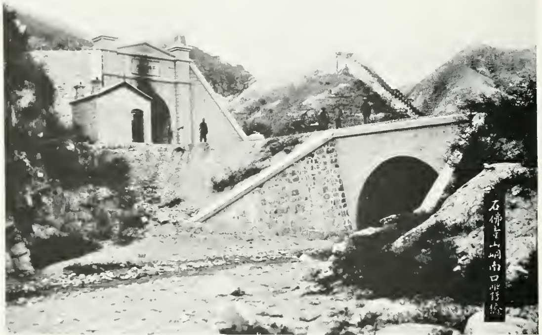
A TUNNEL AND CULVERT ON THE PEKING-KALGAN RAILWAY.
