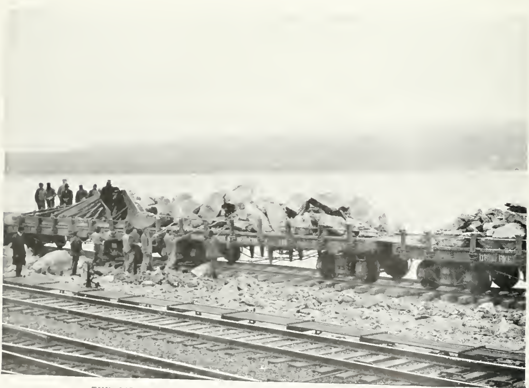
THE LIDGERWOOD UNLOADER DUMPING ROCK FROM A TRAIN, Showing plough and hauling rope.
