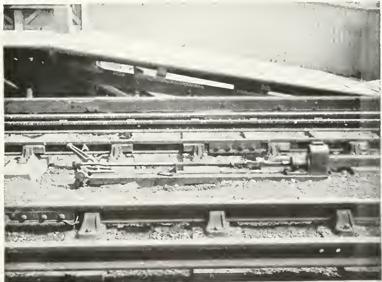
THE AUTOMATIC STOP WHEREBY TRAINS ARE BROUGHT TO A STANDSTILL INDEPENDENTLY OF THE MOTOR IF THE SIGNALS ARE AT DANGER.
