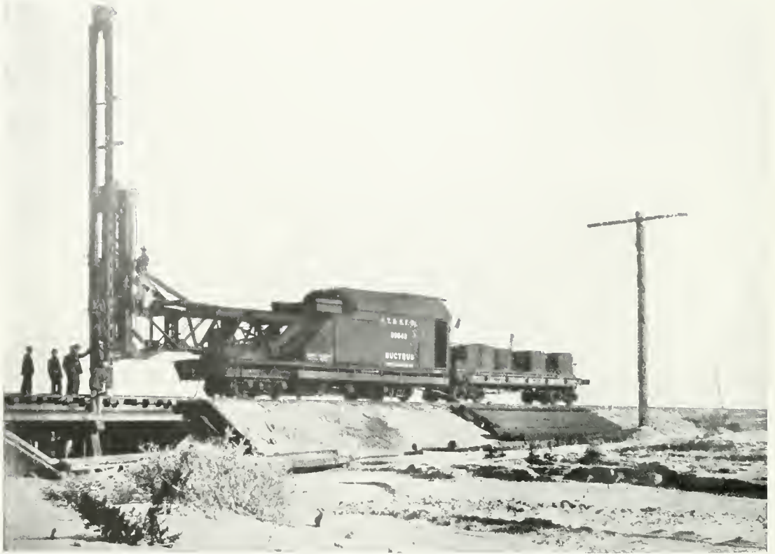
THE BUCYRUS SELF-CONTAINED, SELF-PROPELLING PILE-DRIVER AT WORK UPON THE AMERICAN DESERT.
