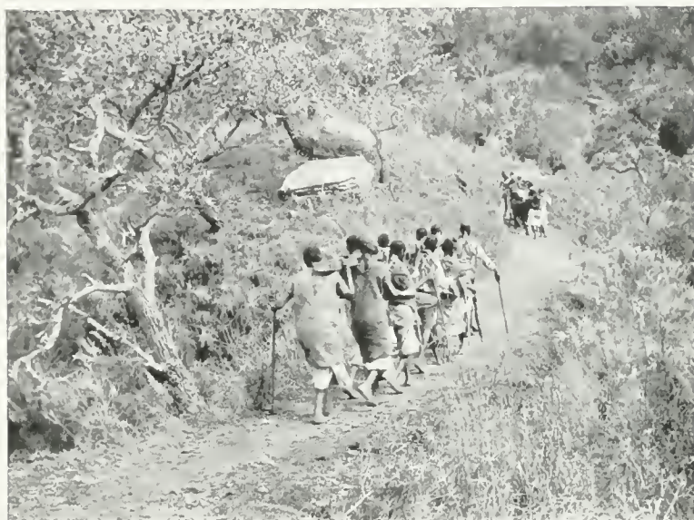
HOW THE HEAVY STEEL PARTS FOR THE PERMANENT WAY WERE TRANSPORTED BY NATIVES TO THE SITE OF ERECTION.
