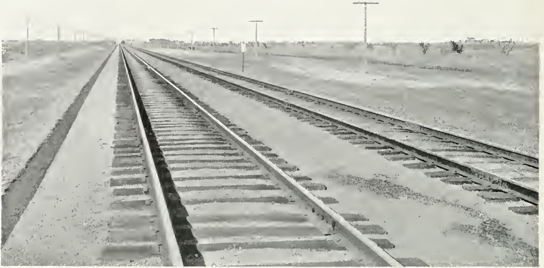
ROAD-BED BALLASTED WITH SHERMAN GRAVEL
