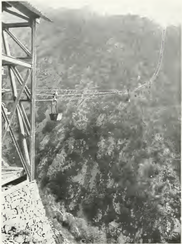
A SPAN OF 1,700 FEET ACROSS A RAVINE IN THE PYRENEES.
