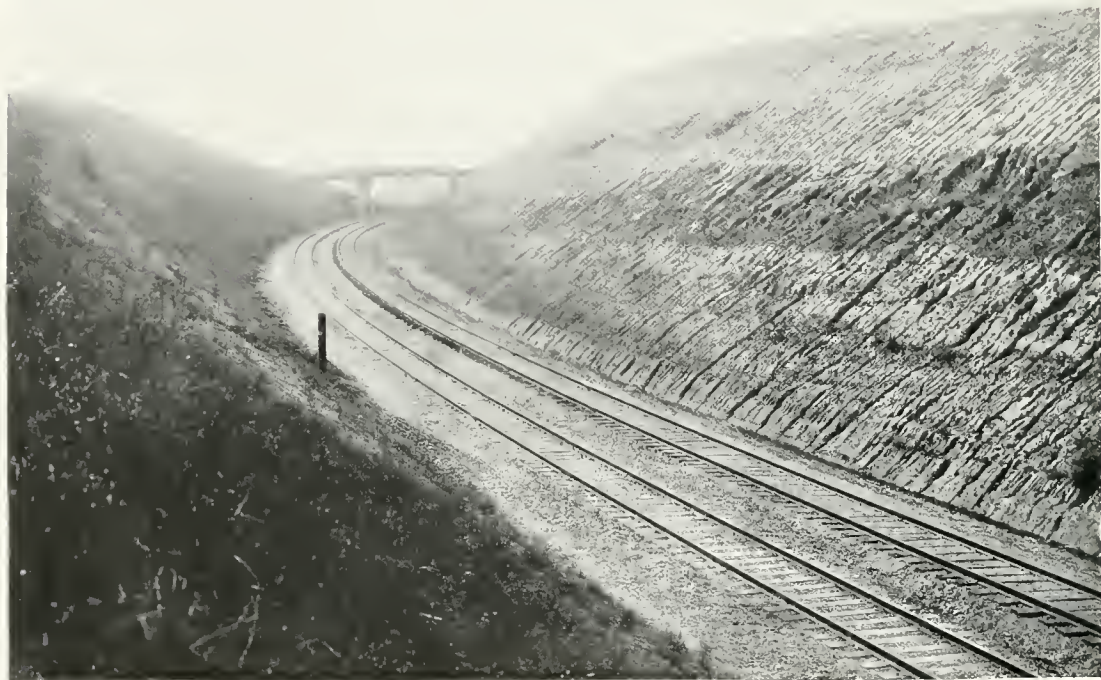
THE BIG CUTTING ON THE LANE CUT-OFF.
