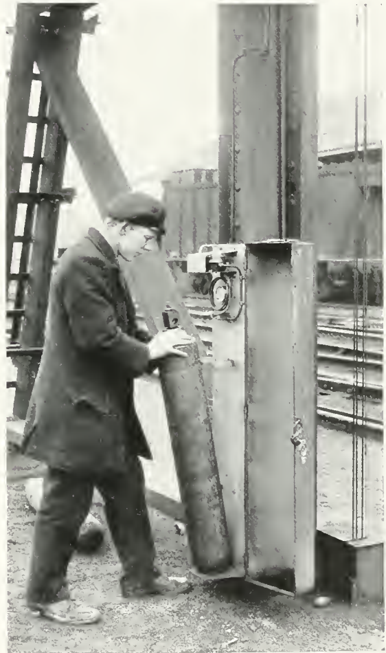
PUTTING IN A FILLED ACCUMULATOR (OLD TYPE OF BOX).
