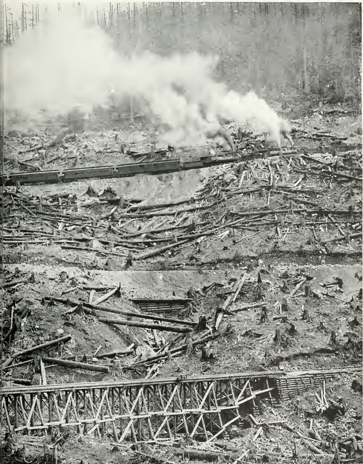
DURING THE PERIOD THE CASCADE TUNNEL WAS UNDER CONSTRUCTION, zig-zag by means of three locomotives. In the photograph four tracks are to be seen. This expensive directly the tunnel was completed.
