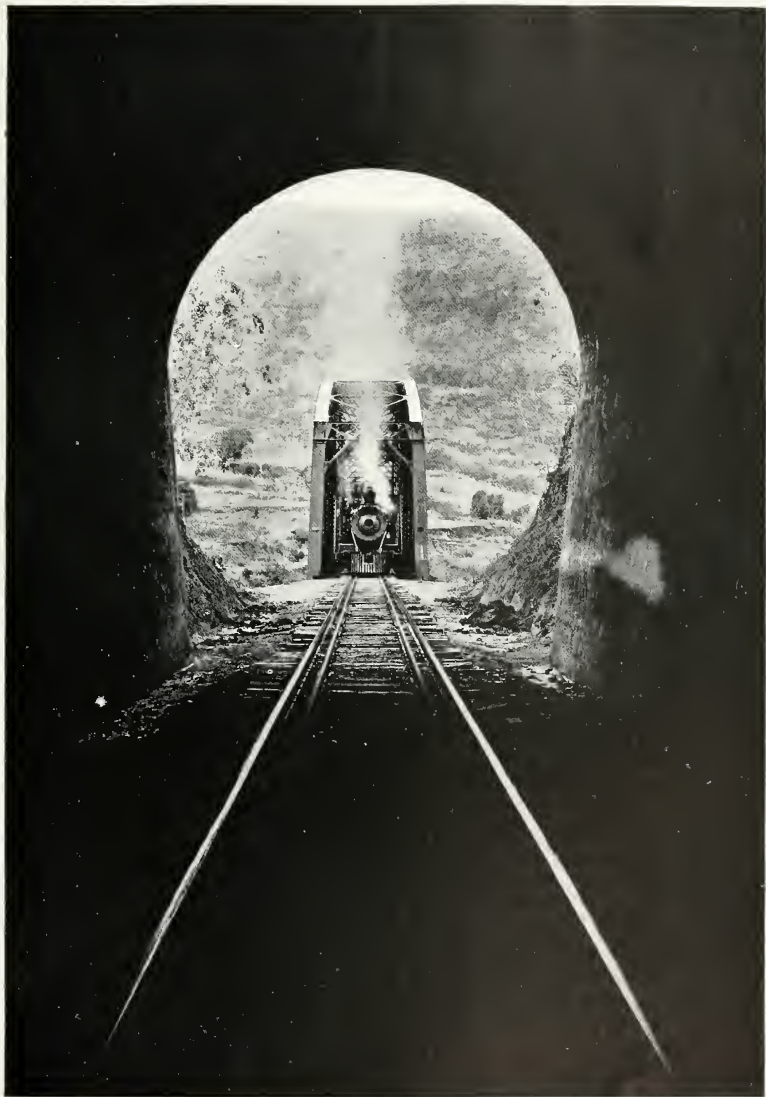
THE FIRST BRIDGE AND TUNNEL SOUTH OF TUXPAN, ON THE TUXPAN-COLIMA BRANCH OF THE NATIONAL RAILWAYS OF MEXICO.
