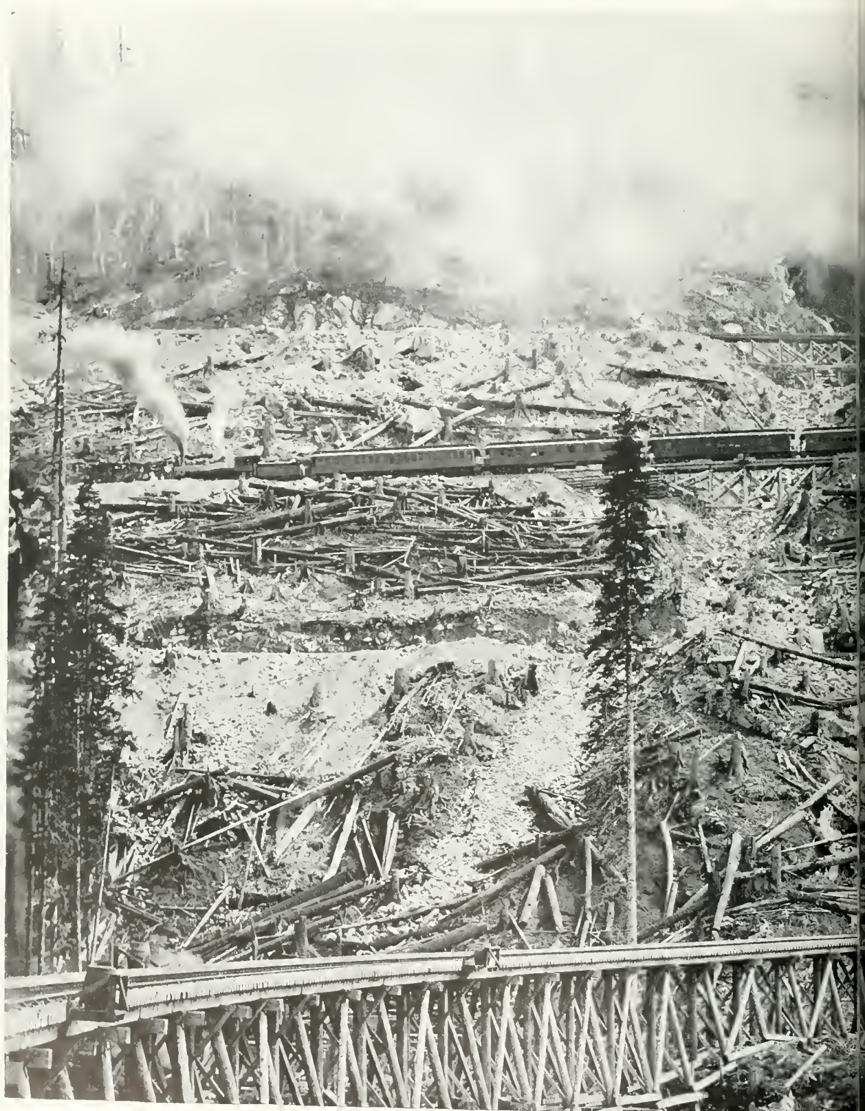
THE "ZIG-ZAG" WHEREBY THE CASCADE MOUNTAINS WERE NEGOTIATED The Great Northern Limited, of seven Pullmans, weighing 280 tons, had to be lifted over the steps of the temporary line was abandoned
