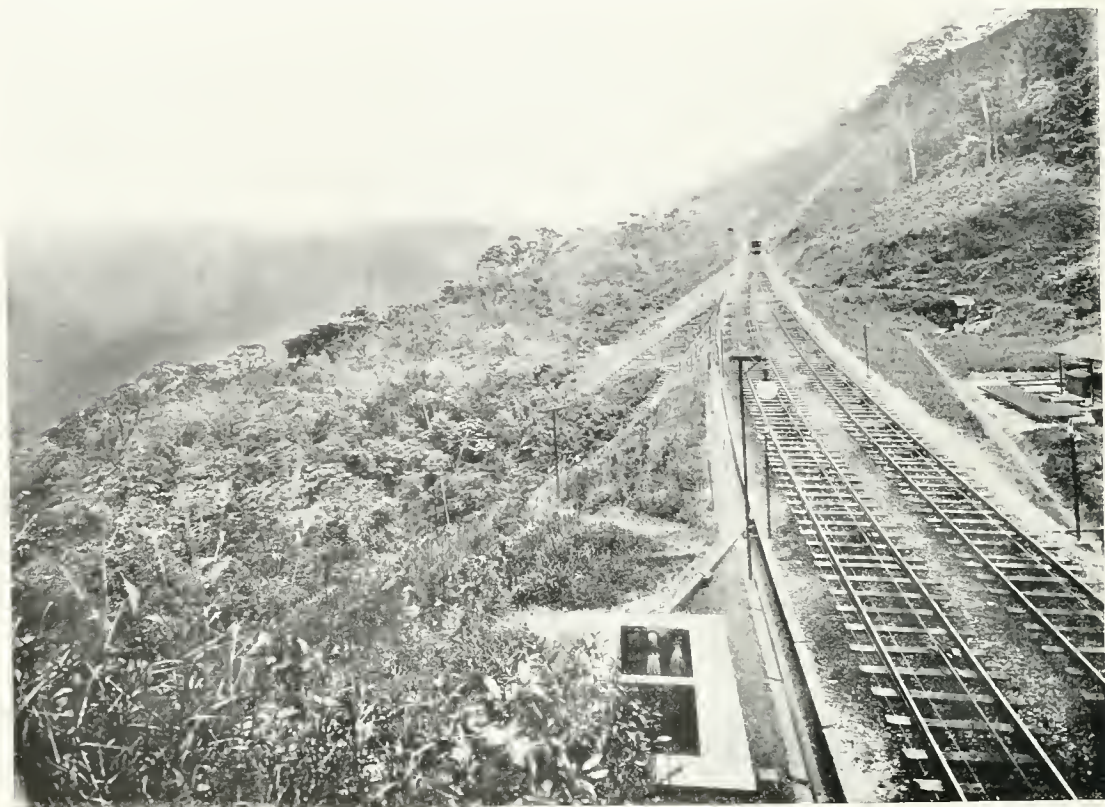
PASSING PLACE ON THE INCLINE, SHOWING UP AND DOWN TRACKS AND CABLES.
