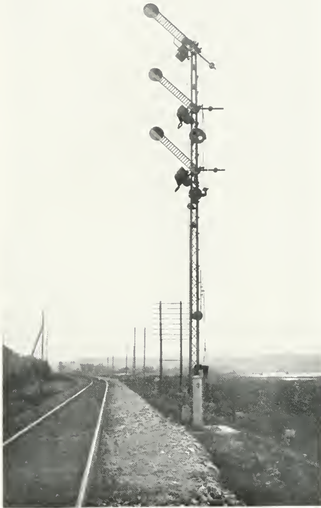
A THREE-ARMED HOME SIGNAL ON THE BERGSLAGENS RAILWAY.
