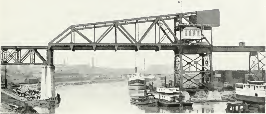
160-FOOT SINGLE-LEAF DOUBLE-TRACK SCHERZER ROLLING LIFT BRIDGE ACROSS THE CUYAHOGA RIVER AT CLEVELAND, OHIO, U.S.A., IN CLOSED POSITION.
