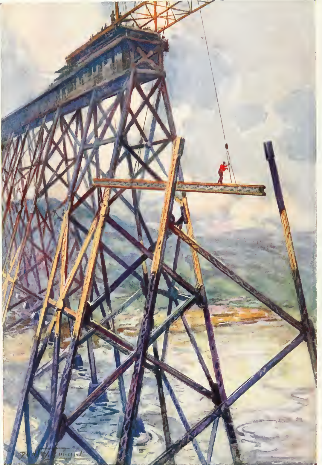
SETTING THE STEEL OF THE BATTLE RIVER VIADUCT OF THE GRAND TRUNK PACIFIC RAILWAY.
