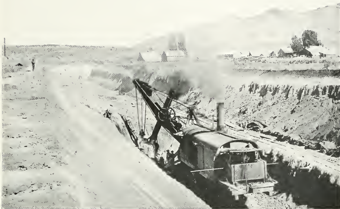
STEAM SHOVEL EXCAVATING THE BOTTOM LIFT OF THE BECKWORTH TUNNEL APPROACH, THE SUMMIT LEVEL OF THE WESTERN PACIFIC RAILWAY, 4,956 FEET ABOVE THE SEA.
