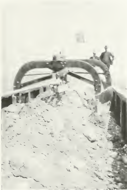
THE BUCYRUS DISCHARGING PLOUGH AT WORK. It is pulled by means of a cable from the extreme rear to the front of the train.
