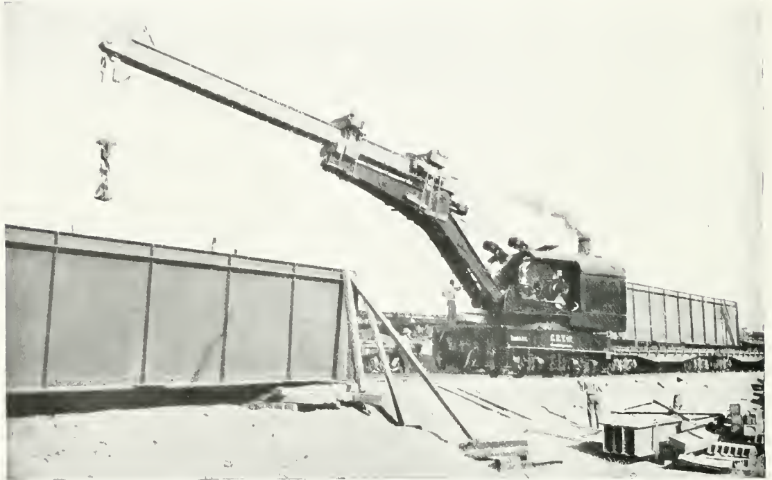
AN INDUSTRIAL WORKS WRECKING CRANE ADAPTED TO HANDLE AN AWKWARD LOAD. An extemporised boom attached to the crane-jib enabled this machine to place unaided an 80-foot girder weighing 20 tons.
