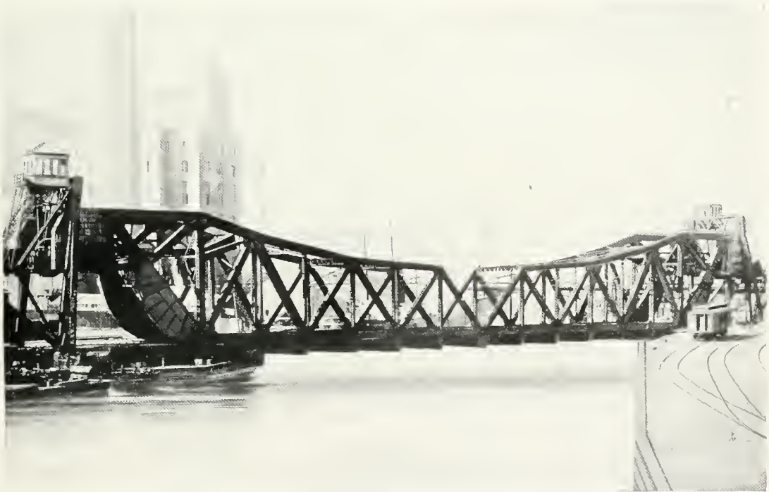
275-FOOT DOUBLE-LEAF DOUBLE-TRACK SCHERZER ROLLING LIFT BRIDGE ACROSS THE CHICAGO RIVER AT THE ENTRANCE TO THE GRAND CENTRAL STATION, CHICAGO.
