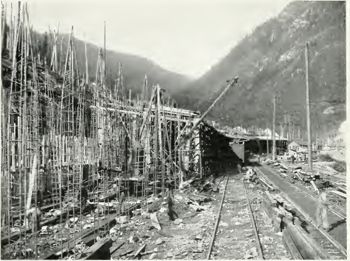
NEW CONCRETE SNOW-SHED, CASCADE SUMMIT.
