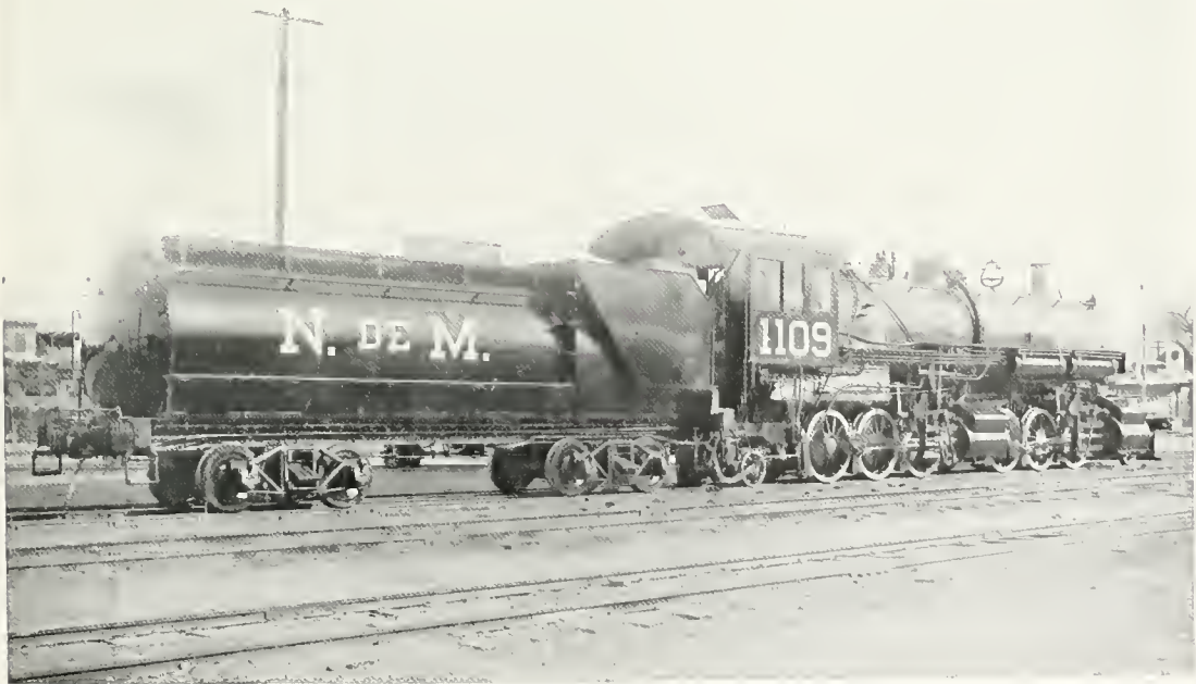
ANOTHER VIEW OF THE GIANT MALLETT LOCOMOTIVE. The tender carries 7,500 gallons of water, and 3,300 gallons of oil.
