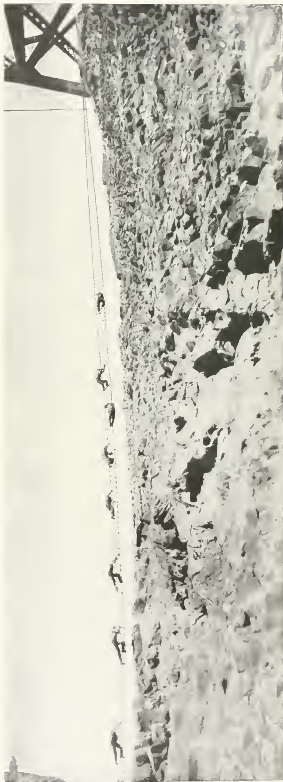
HOW THE "FLIES" WHO BUILT THE CROOKED RIVER CANYON BRIDGE REACHED THEIR WORK. A rope ladder was slung over the cliff communicating with the camp below.
