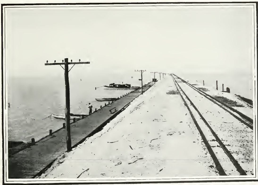
THE FINISHED EARTHEN EMBANKMENT IN THE "SHALLOWS" BETWEEN THE KEYS—AS SOLID AS A ROCK
