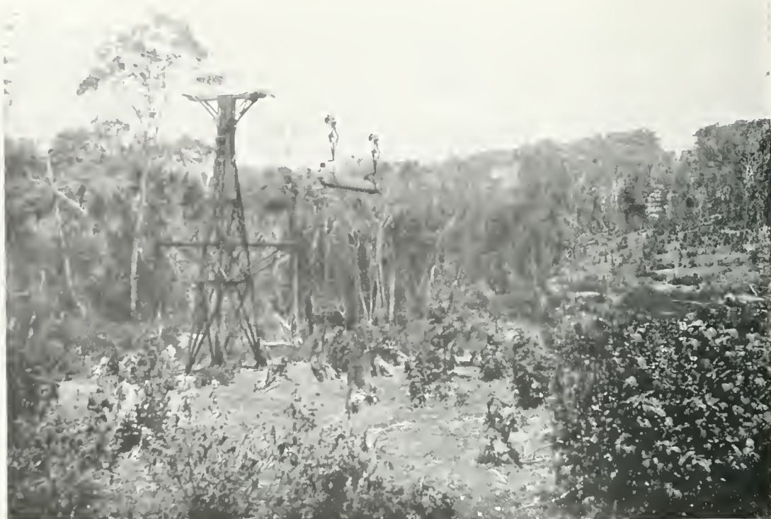
THE RISE FROM THE UPPER STATION TO THE EDGE OF THE PLATEAU ON THE USAMBARA AERIAL RAILWAY.
