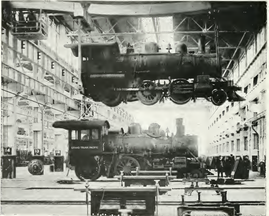
SLINGING A 100-TON LOCOMOTIVE.
