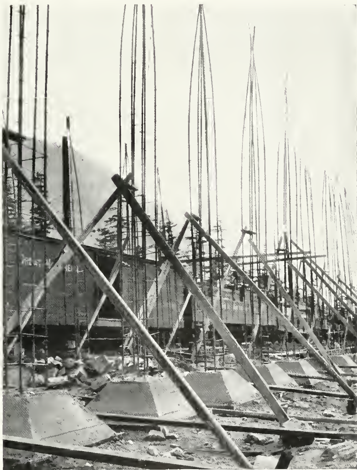
THE NEW CONCRETE SNOW-SHEDS, CASCADE SUMMIT. The reinforcing steel for the posts on the lower side of the line.
