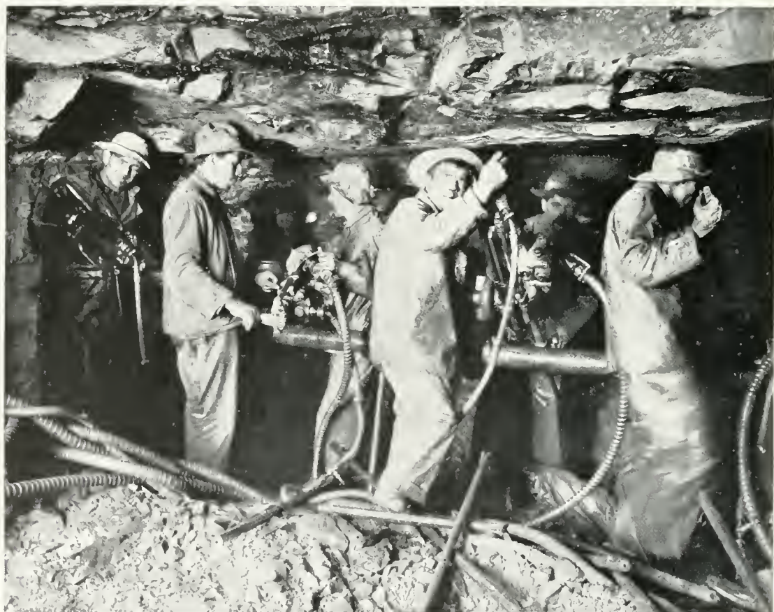
Photograph by permission of the Canadian Northern Railway. DRIVING THE TUNNEL THROUGH MOUNT ROYAL TO GIVE THE CANADIAN NORTHERN ACCESS TO MONTREAL.
