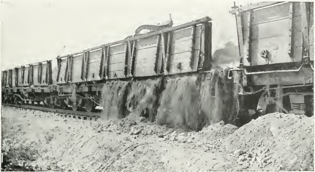
THE SPOIL FALLING FROM THE TRUCKS AS THE UNLOADER IS PULLED ALONG. The sides of the Truck are top-hinged doors.
