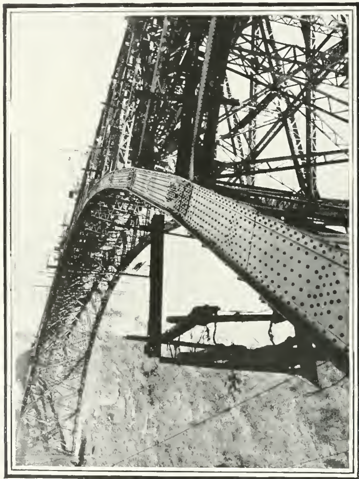
THE ARCH OF THE VICTORIA FALLS BRIDGE FROM BENEATH DURING CONSTRUCTION.
