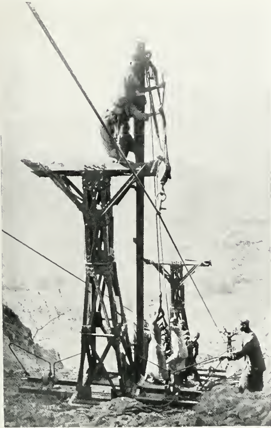
LIFTING THE CABLES UPON THE SUPPORTS.
