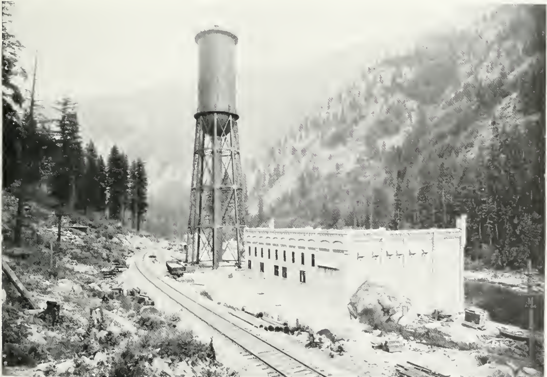
THE POWER-HOUSE IN THE TUMWATER CANYON.
