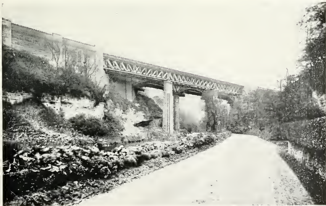
MILLER'S DALE VIADUCTS. 1905.
