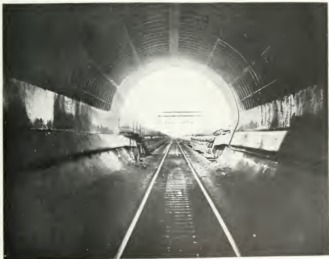
THE ST. CLAIR TUNNEL.
