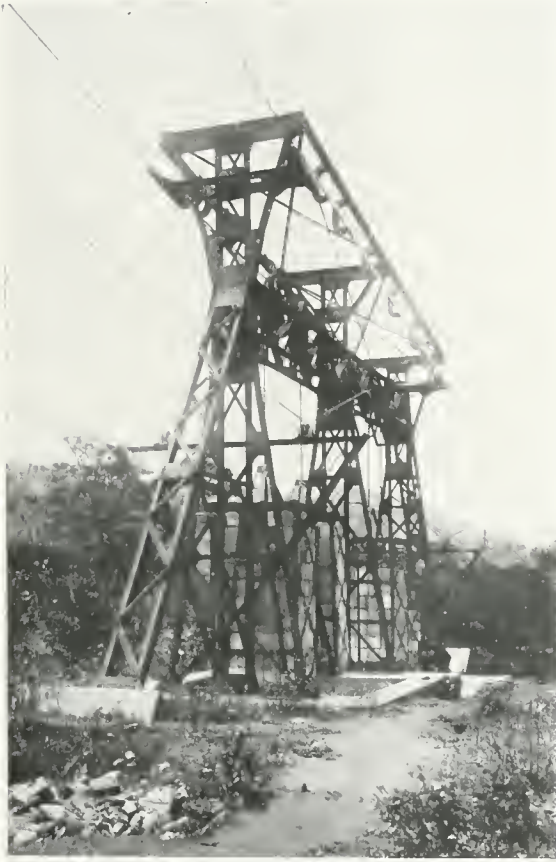
A TENSION STATION, SHOWING THE TOWERS WITH THE CONCRETE BLOCKS WHEREBY THE LINE IS KEPT TAUT.
