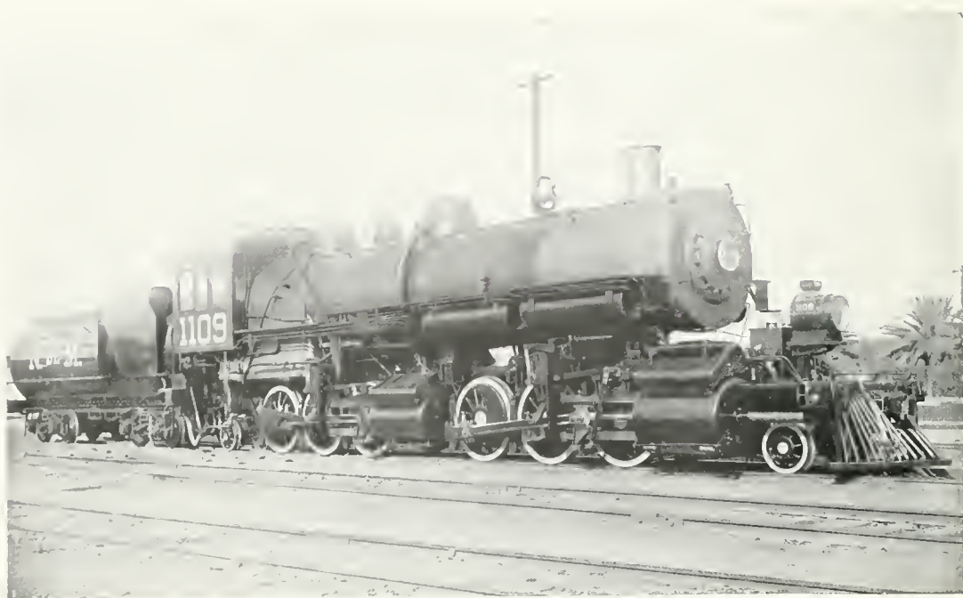
NATIONAL RAILWAYS OF MEXICO'S MALLET ARTICULATED COMPOUND OIL-BURNING FREIGHT LOCOMOTIVE.
