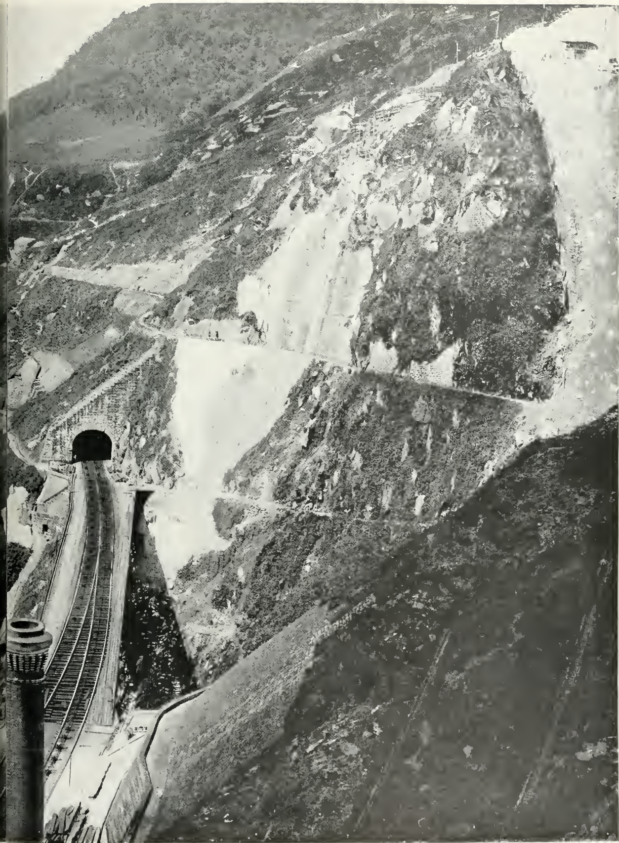
Photograph by courtesy of the San Paulo Railway.
