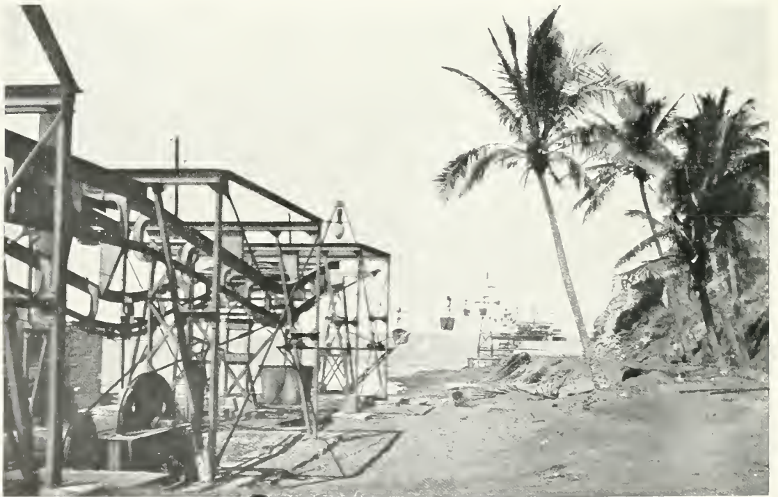
THE NICKEL ORE AERIAL RAILWAY IN NEW CALEDONIA.
