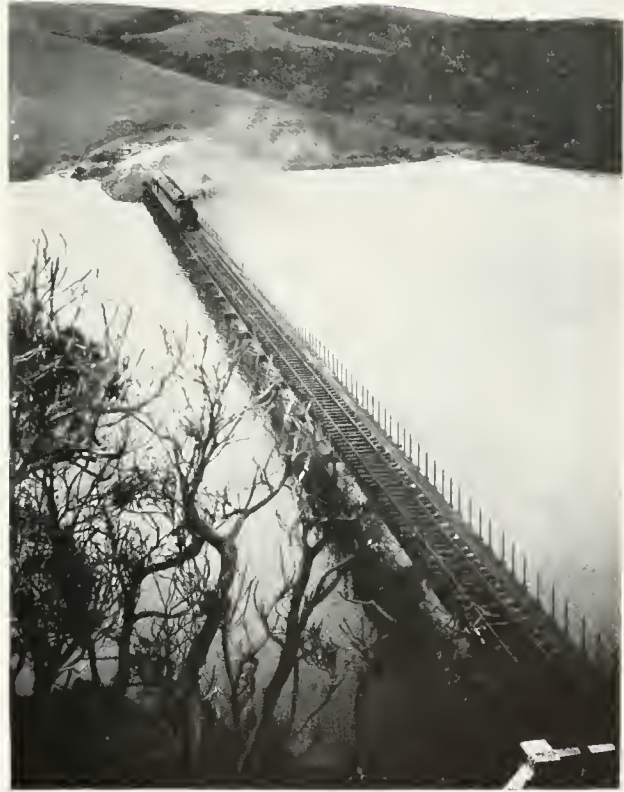
Photograph supplied by the South African Railways. EXPRESS CROSSING THE IFAFA BRIDGE, NATAL.
