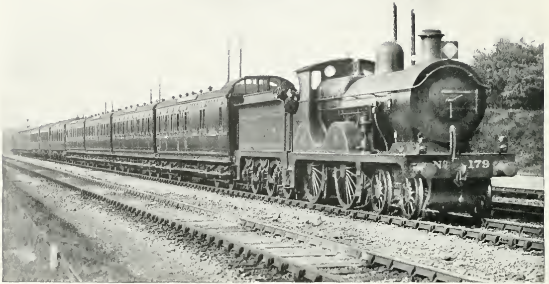
THE SOUTH EASTERN FOLKESTONE-BOULOGNE BOAT EXPRESS. DRAWN BY 4-4-0 LOCOMOTIVE, AND WITH LOAD OF 320 TONS, MAKING 50 MILES AN HOUR.
